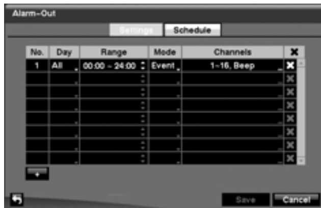
Figure 3-42 Alarm-Out Schedule Screen
